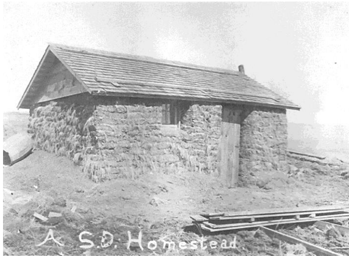
Sod house in South Dakota.
